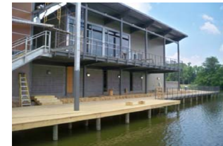
Multi-Purpose Building - Greenwood
