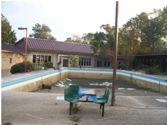
Pool Prior To Demolition
