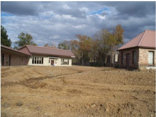
Site After Pool Removal
