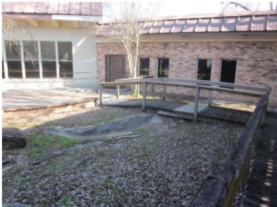
'Blue Room' Prior To Demolition
