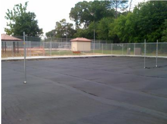
Sand Volleyball During Construction
